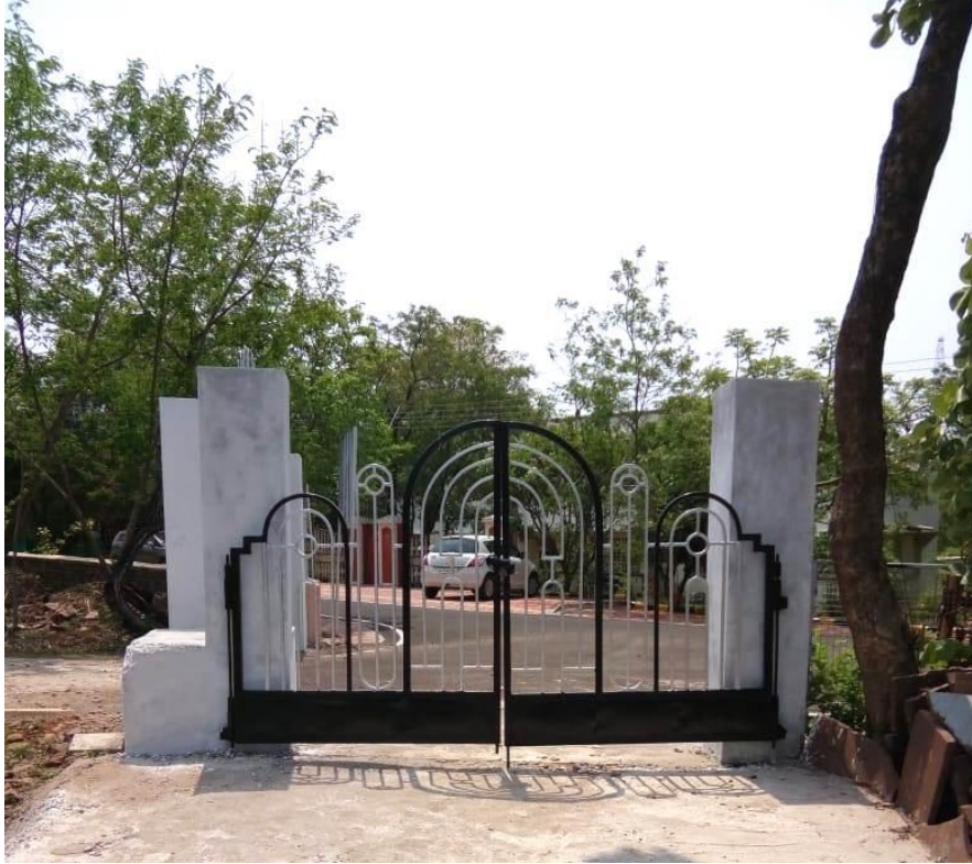
Newly constructed gate in the science park
